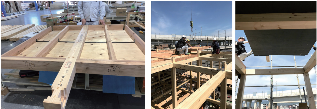
Fig. 11 Factory fabricated panels and during erection
