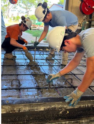
a) Concrete Placement of Longitudinal Panel Joint
