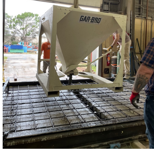
b) Concrete Placement of Transverse Panel Joint
