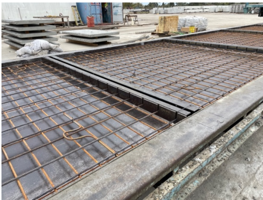
a) PCP Reinforcement
