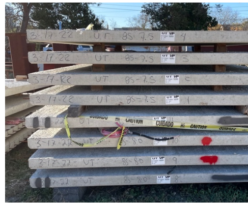
b) Finished PCPs
