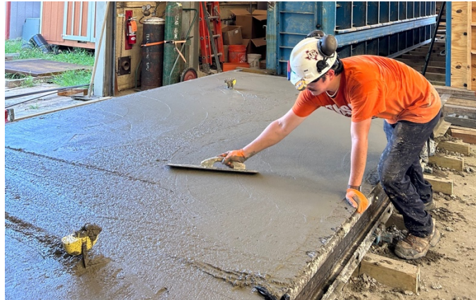
c) CIP Layer Placed and Finishing
