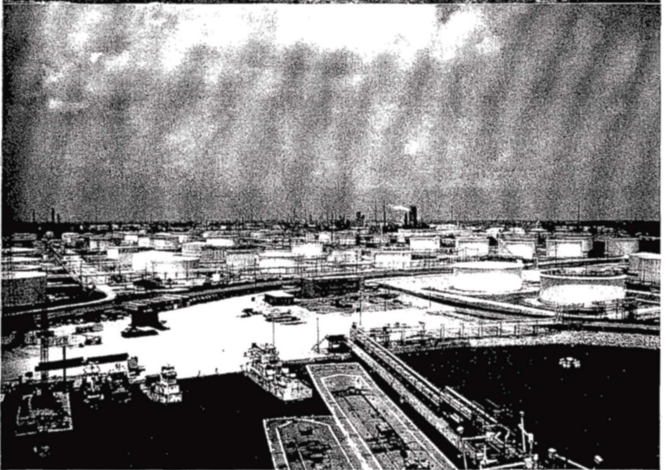
Figure 2. Examples of coastal structures (a) exposed vertical seawall at Galveston with riprap and piers, and (b) typical port facilities with bulkheads and riprap such as this refinery at Baytown.
