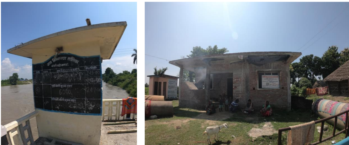
Figure 30: left image: the blackboard at the Kosi River barrage stating river discharge, which was barely understandable; the Right image evacuation shelter which could barely fit four people, prepared for the whole ward by an NGO, which had a board written “Local Disaster and Climate Change Resilient Emergency Shelter”, built at the cost of 2,258,468.55 NRs which is approximately £14,150.
