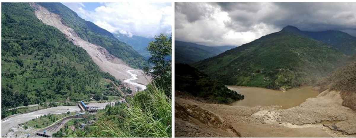
Figure 18: left image showing landslide of Jure blocking the Sunkosi River, Right Image Showing dam formed by landslide. (Source: Panthi 2021)
