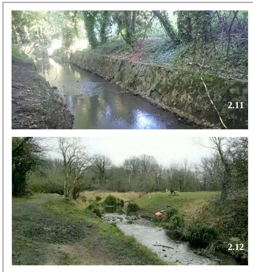
Figure 2.11. Photograph of the restored Hogsmill River site at Green Lanes; Figure 2.12 Photograph of the unrestored Hogsmill River site at Green Lanes.
