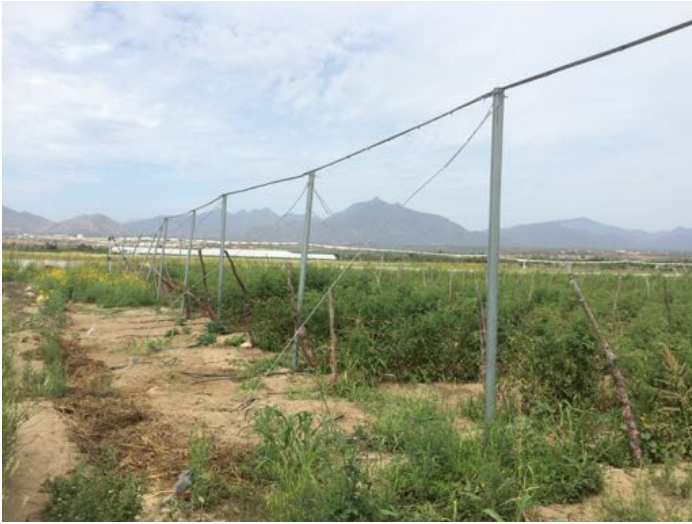
Destroyed Infrastructure farms in Baja California Sur, Mexico
