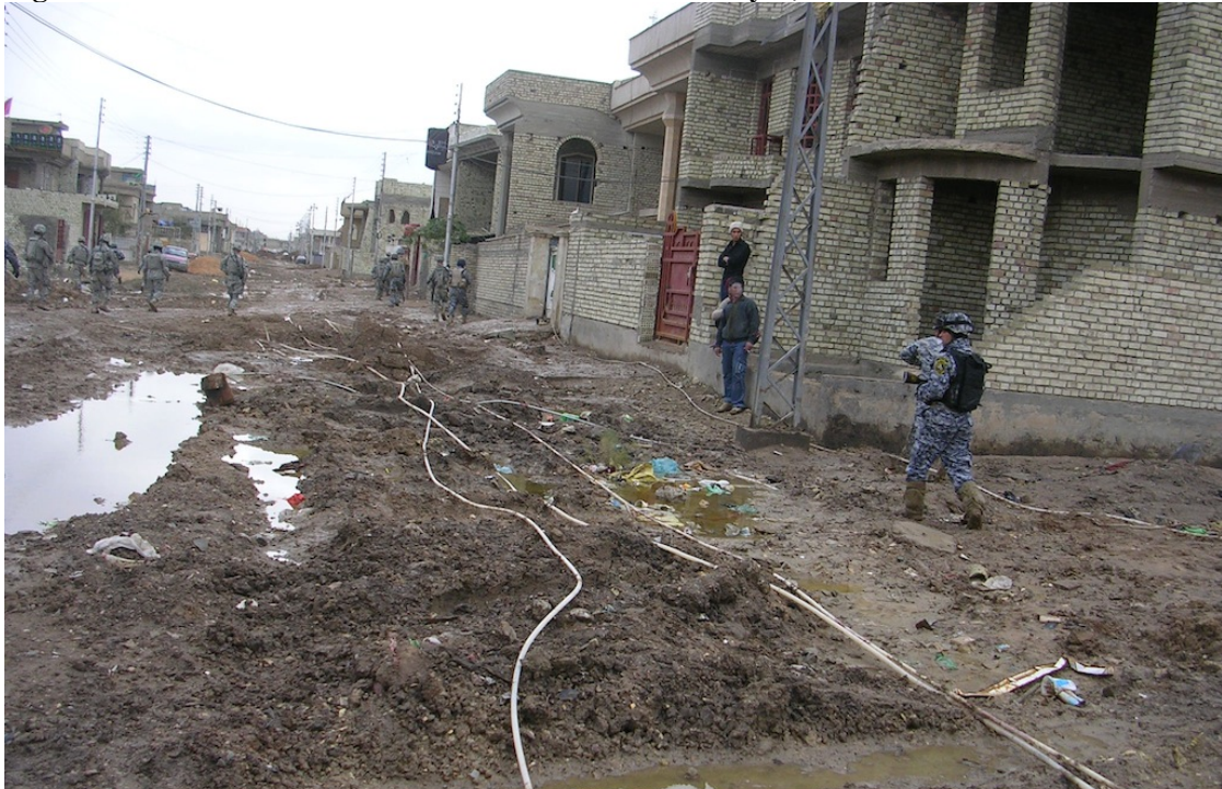
Figure 5.3 – New Construction in Southwestern Beladiyat, 2008
