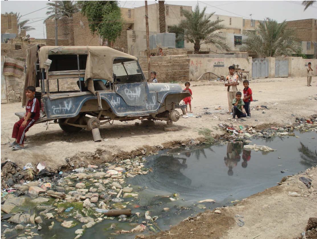
Figure 6.2 – Open Sewers in Central Kamaliyah
