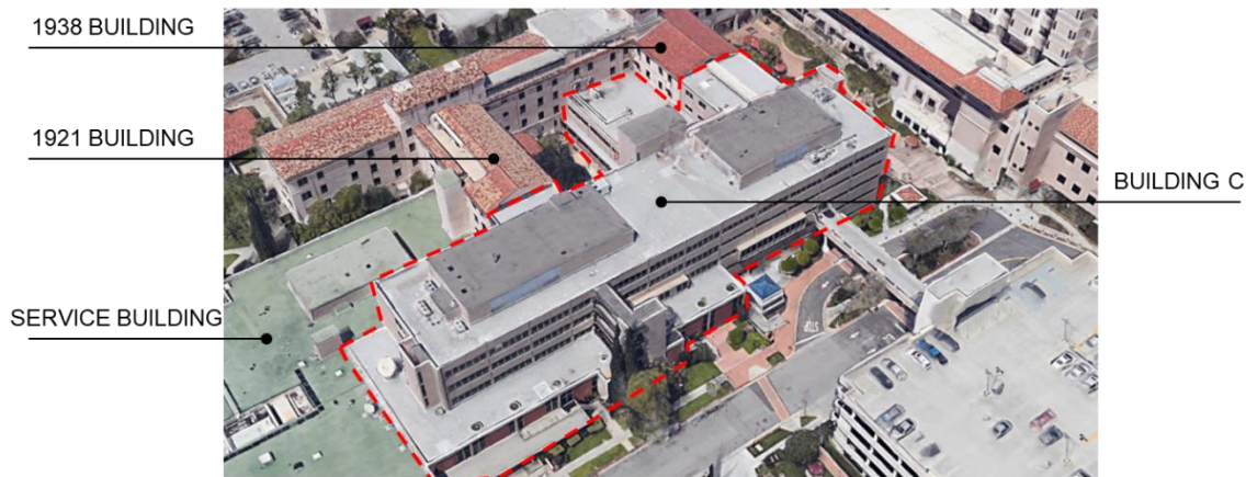
Figure 2.24. General localization of building C.
