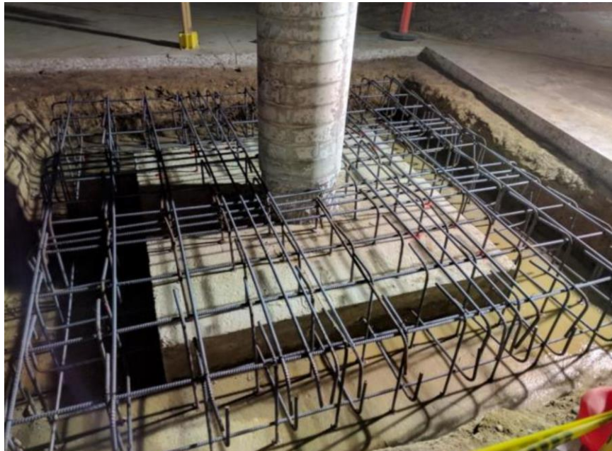
Figure 2.42. Increasing in the size of the foundation of one column.
