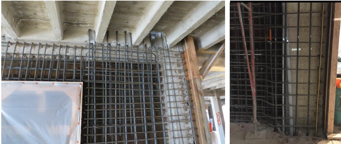
Figure 2.58. Construction of shear walls
