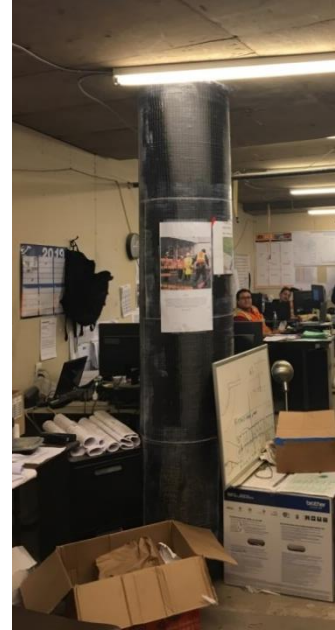
Figure 2.46. FRP strengthening of circular column in the basement
