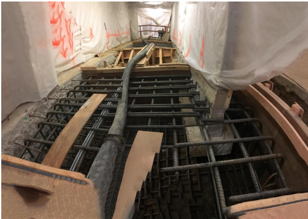
Figure 2.37. Construction of the new footing with the existing footing embedded
