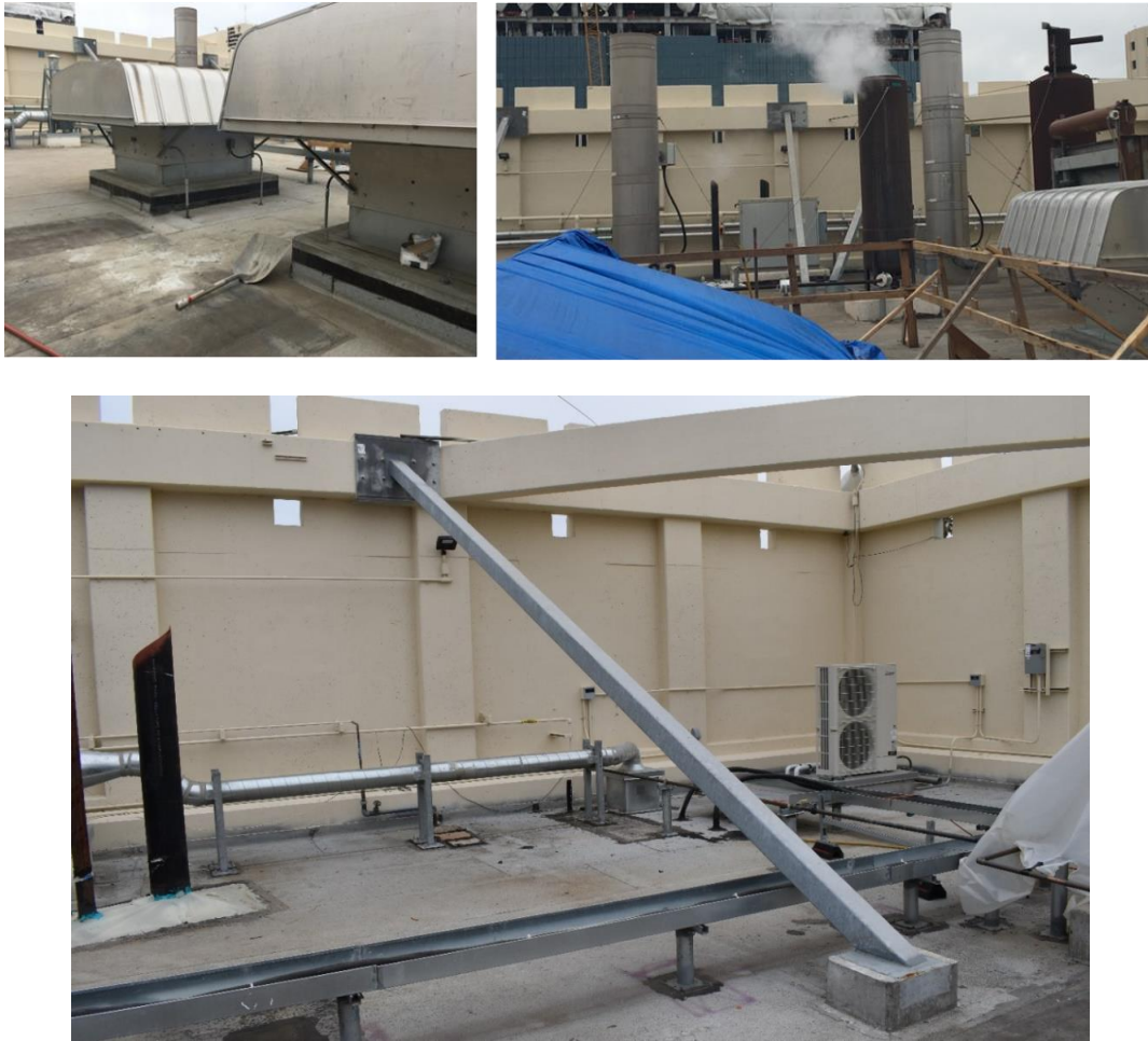
Figure 2.19. Works on the roof: Equipment bolted to the slab (top left), cable bracing of pipes in cantilever (top right) and bracing of parapets with diagonal elements (bottom).
