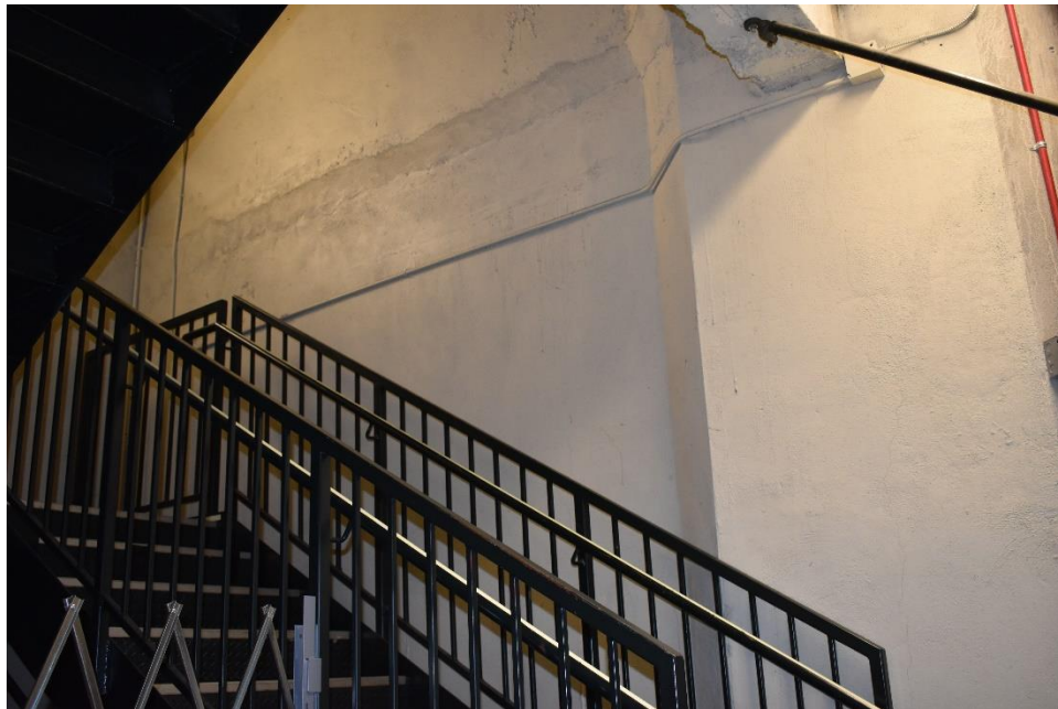
Figure 2.57. View of Shear Wall E1
