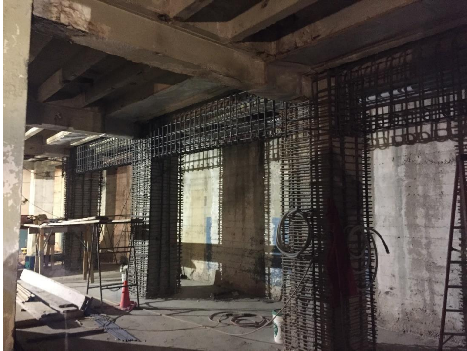
Figure 2.56. Jacketing of columns
