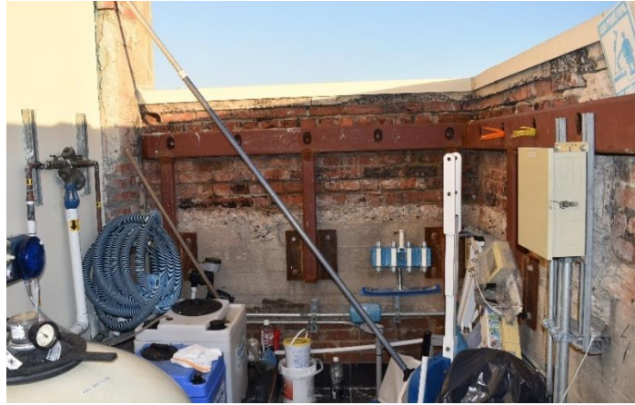
Figure 2.60. Parapet bracing
