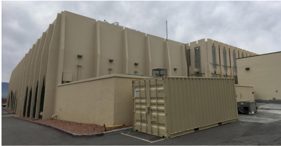
Figure 2.11. General view of the power plant: chiller facility (left building) and steam plant (right building)
