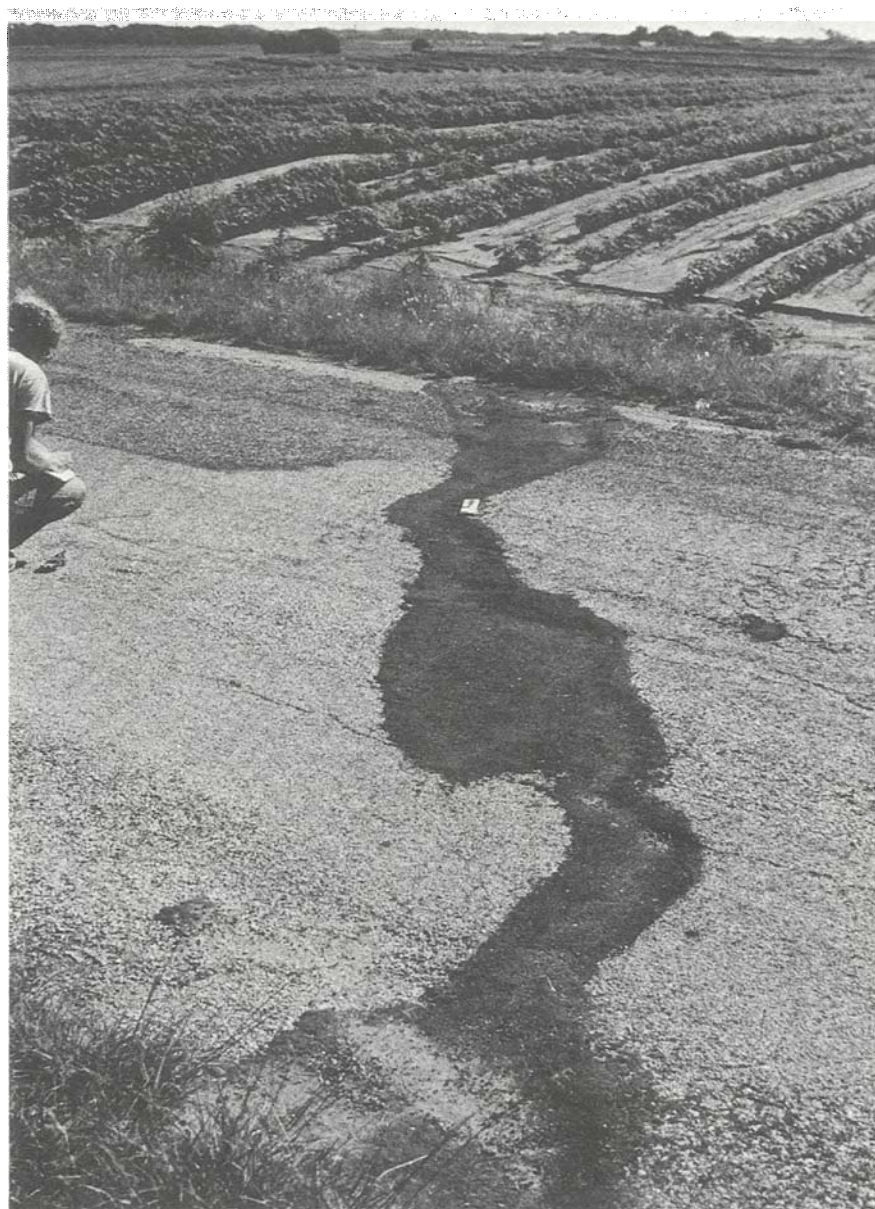
Figure 28. Microfault across County Road 2639 in central Hall County. Left side of the fracture is depressed 3 to 4 cm relative to right side. Fault continues about 30 m into cultivated field.
