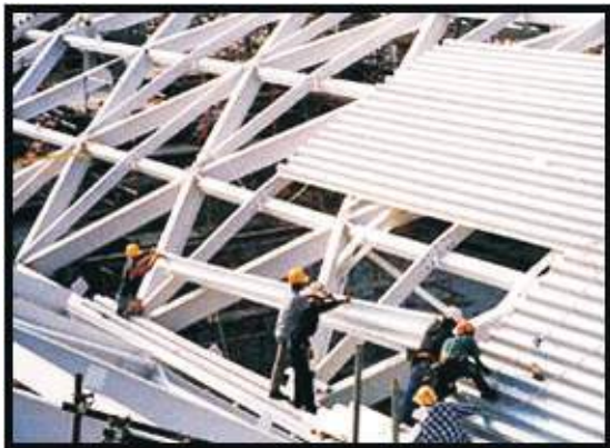
Gambar 11. Proses pemasangan lembar atap di Chek lap kok Airport
