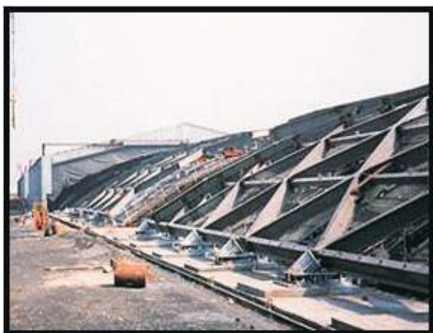
Gambar 7. pemasangan rangka atap di Chek lap kok Airport
