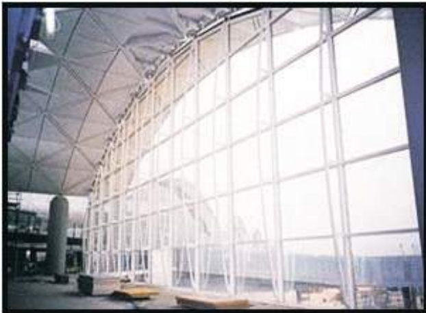
Gambar 19. dinding curtain
