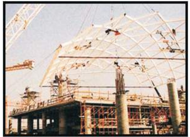
Gambar 8. Proses pemasangan rangka atap di Chek lap kok Airport
