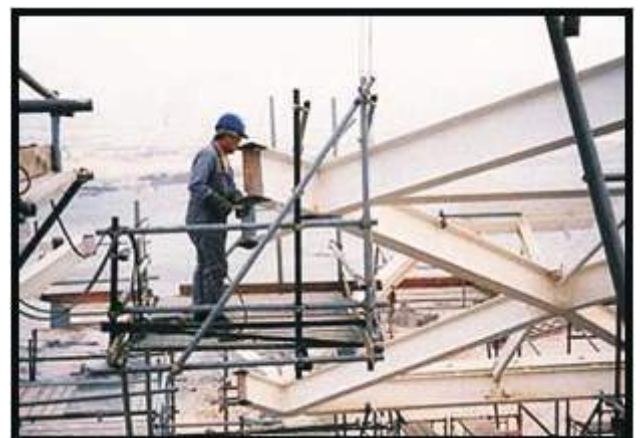
Gambar 9. Proses pemasangan rangka atap di Chek lap kok Airport
