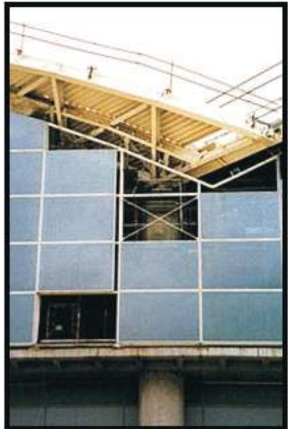
Gambar 17. dinding curtain
