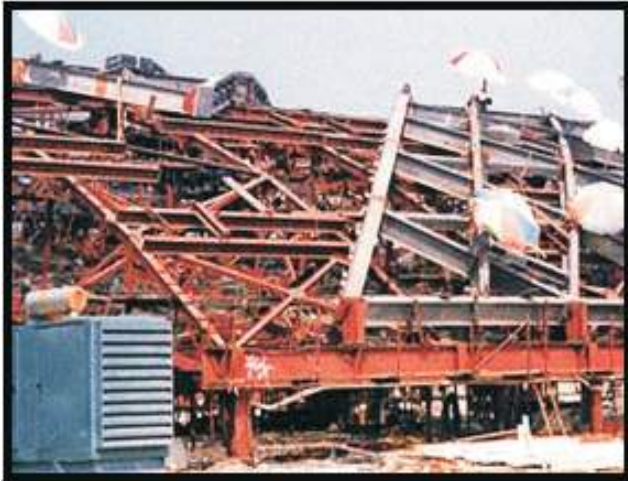
Gambar 6. Proses pemasangan rangka atap di Chek lap kok Airport
