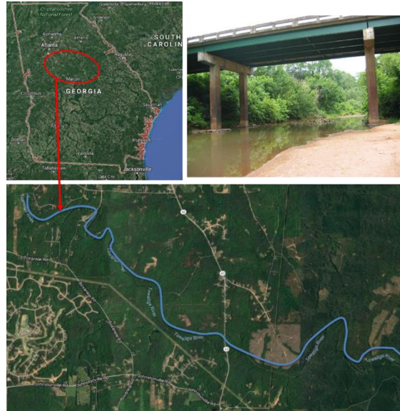
Figure 3.2. Location and view of Towaliga River Bridge
