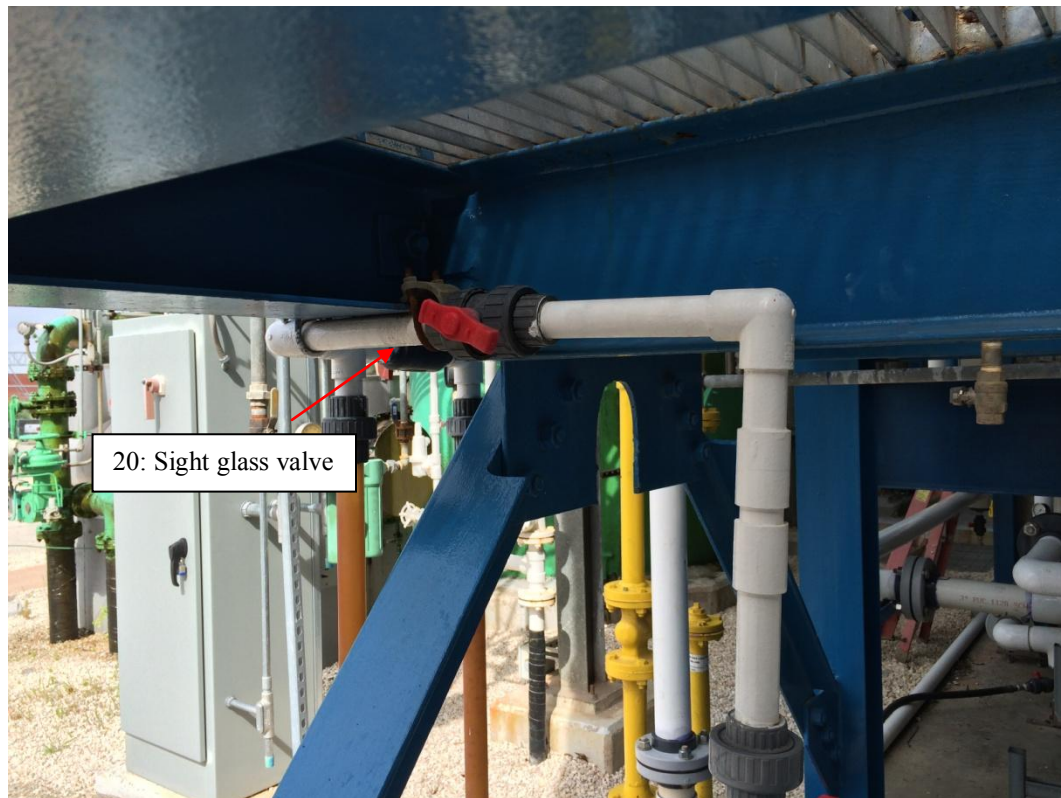
Figure B-9: MicroMotion outlet flow associated valve.
