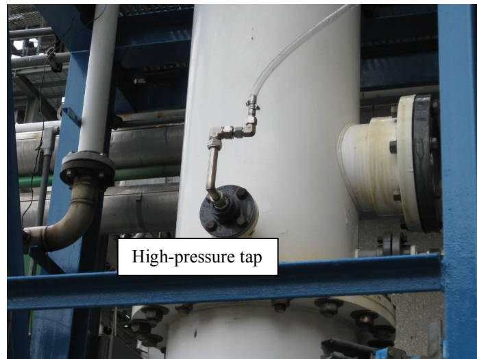
Figure B-13: Column mid-section.
